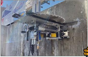
S-300H hydraulic wall saw with electric feed system consisting of S-070 hydraulic motor 550rpm for 30-36" blades with USA flush pattern, track rail 1200mm x qty-2 and 600mm x qty-1, SA0207 feed motor (same track, feedmotor and control box as SS-300R), AP-3300 control box, plunge cutting blade guard 30" (for larger blade guard use 152128), and joint plate & screws
